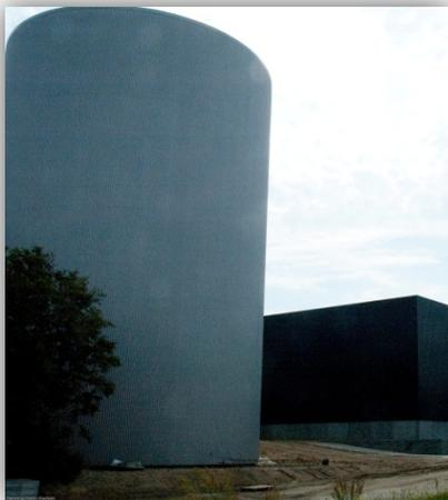
10 MW. The water table of the tank is elevation 85 and keeps the pressure in the entire district heating system.
